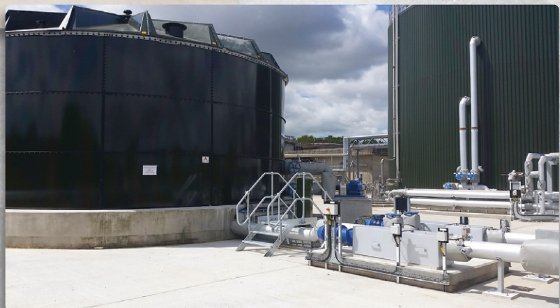
Sludge blending tank - Courtesy of Nomenca
