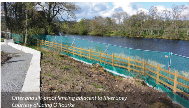
Balancing pond / Silt control from dewatering excavations Courtesy of Laing O'Rourke
