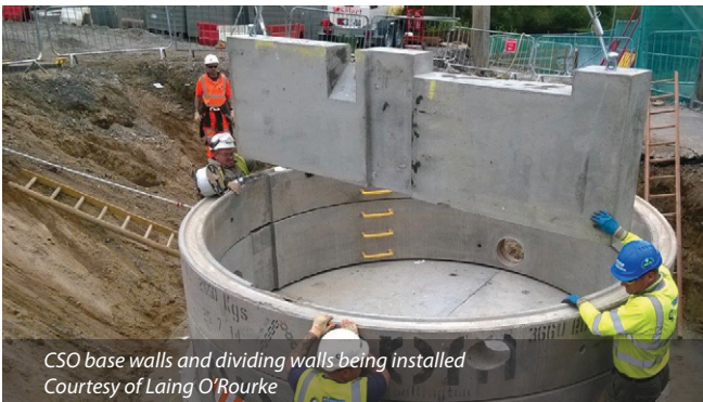
Precast CSO base installation - Courtesy of Laing O'Rourke
