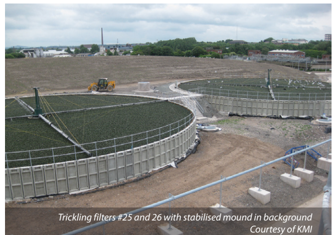
Humus tanks #06, 07 and sludge holding tank - Courtesy of KMI
