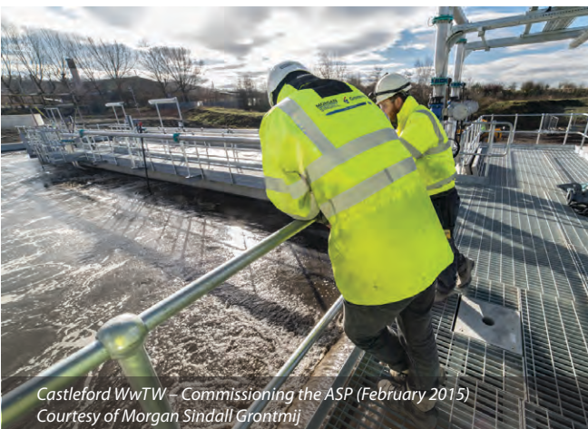
Installation of poly dosing system (March 2015) Courtesy of Morgan Sindall Grontmij
