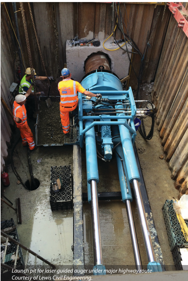
Full depth shaft construction - Courtesy of Lewis Civil Engineering
