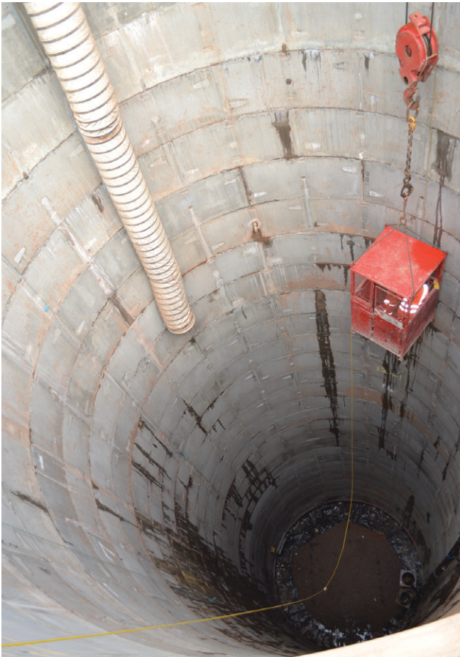
Full depth shaft construction - Courtesy of Lewis Civil Engineering
