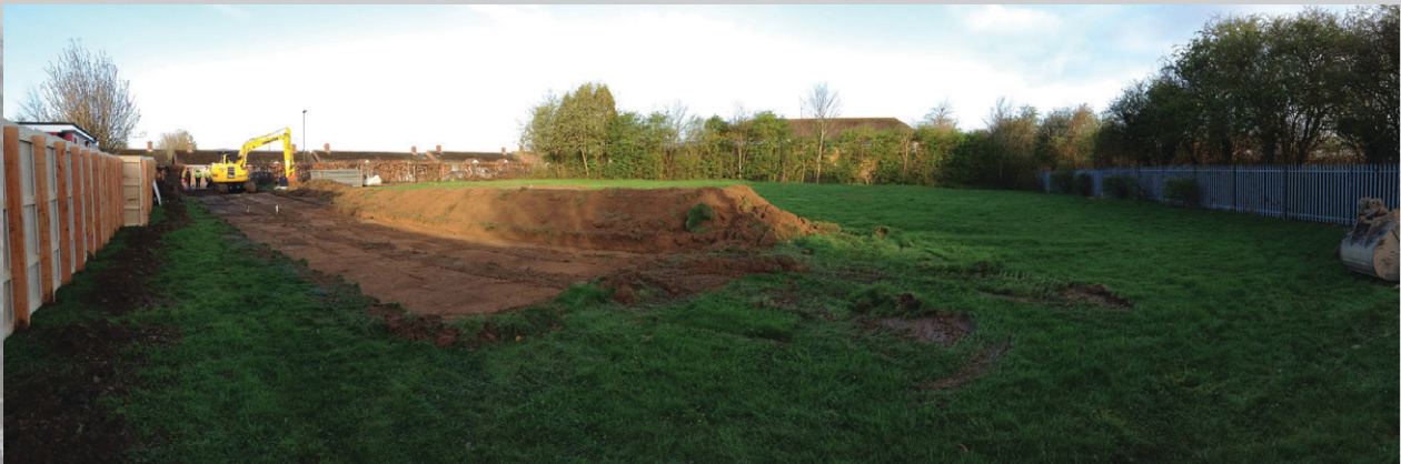
(Above) Site stripping (Below) Site compound following establishment. A secure and self-contained site was required Courtesy of Lewis Civil Engineering
