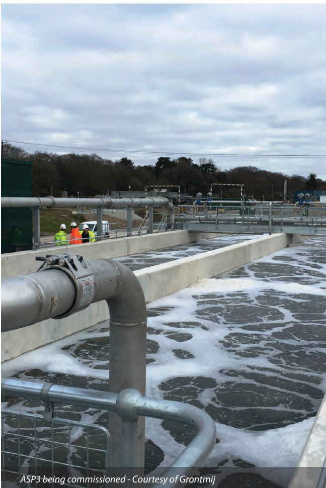
ASP3 structure being water tested - Courtesy of WECS Civils
