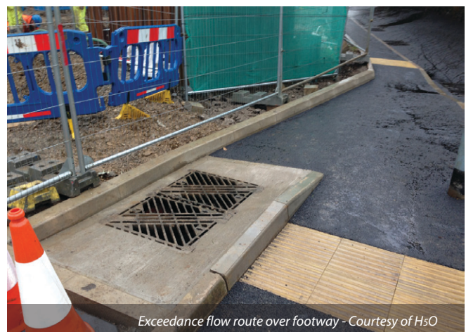
New torrent gratings on Boringdon Hill in operation - Courtesy of H5O
