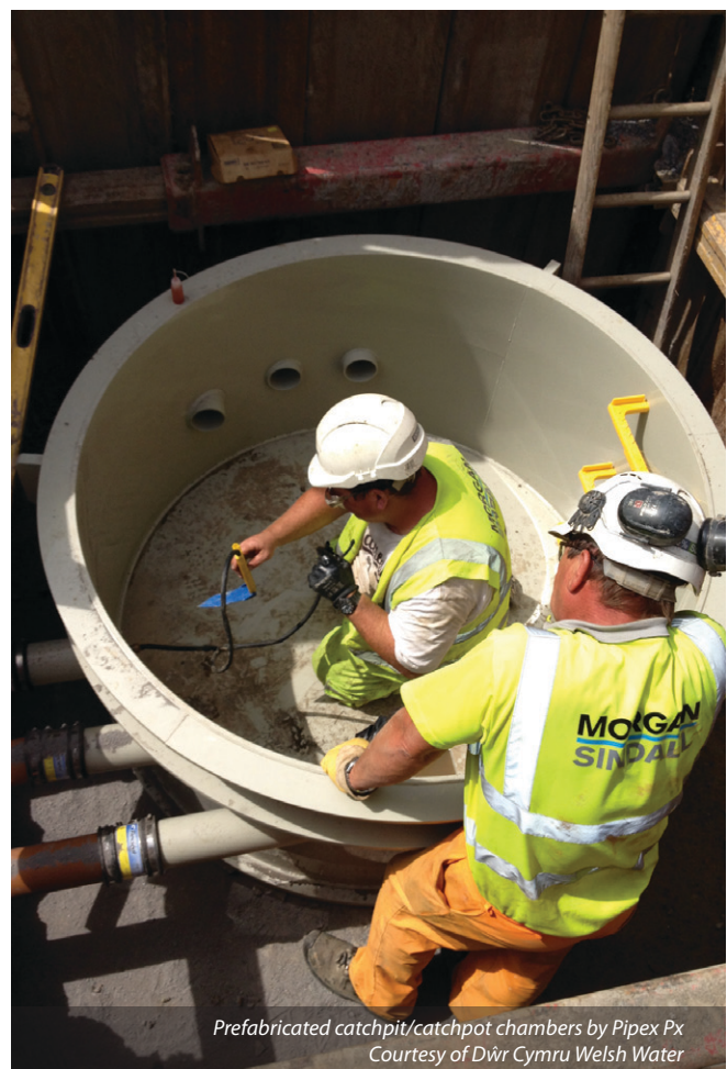
Kijlstra precast MCC chamber being lifted into place at Gowerton WwTW - Courtesy of Dŵr Cymru Welsh Water
