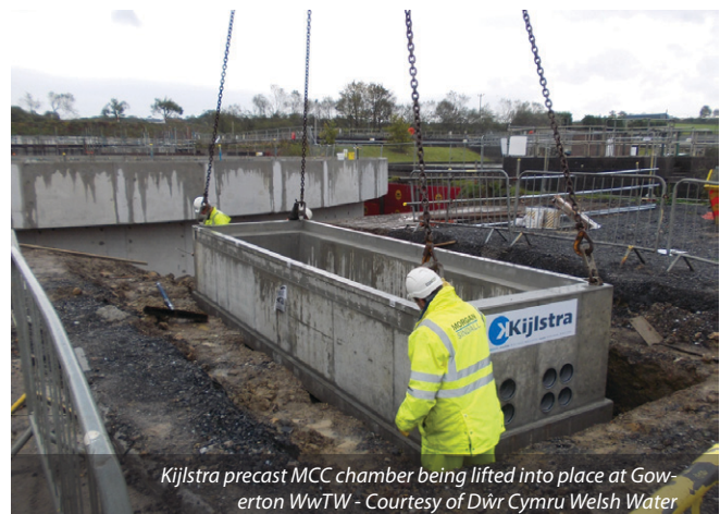
Temporary works at Gowerton WwTW Courtesy of Dŵr Cymru Welsh Water
