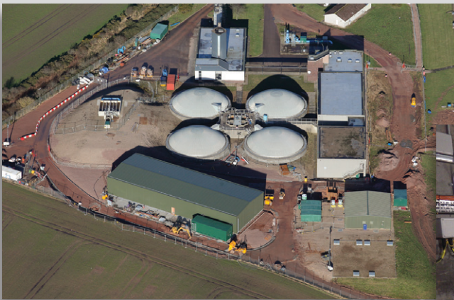
Aerial photo of Forehill WTW - Courtesy of Laing O'Rourke
