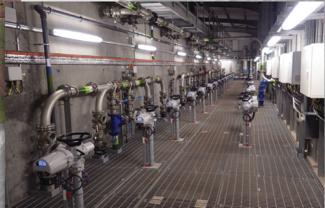
DfMA pipe module successful installation - Courtesy of Laing O'Rourke
