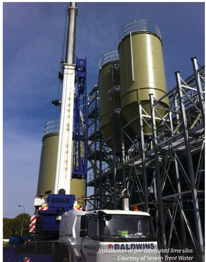
Installation of pre-fabricated lime silos
