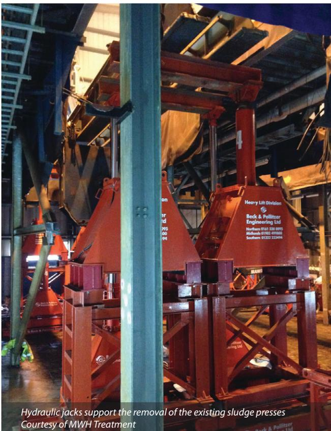
Hydraulic jacks support the removal of the existing sludge presses
