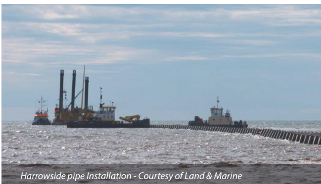
Harrowside pipe Installation - Courtesy of Land &amp; Marine
