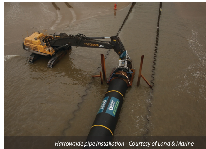
Harrowside pipe Installation - Courtesy of Land & Marine
