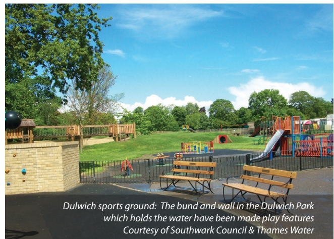
Dulwich Park - retaining wall Courtesy of Southwark Council & Thames Water
