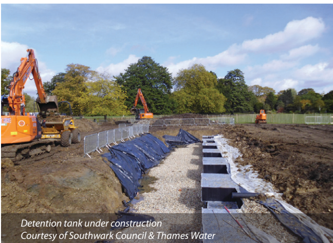
Detention tank under construction Courtesy of Southwark Council & Thames Water
