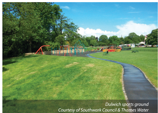
Dulwich sports ground: The bund and wall in the Dulwich Park which holds the water have been made play features Courtesy of Southwark Council & Thames Water
