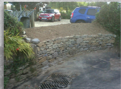
Completion of garden wall Courtesy of HsO
