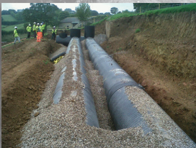
Welding team on site following install Courtesy of HsO
