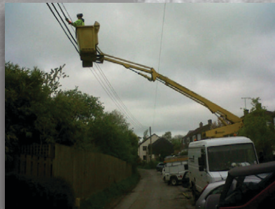
Shroding of overhead by WPD Courtesy of HsO
