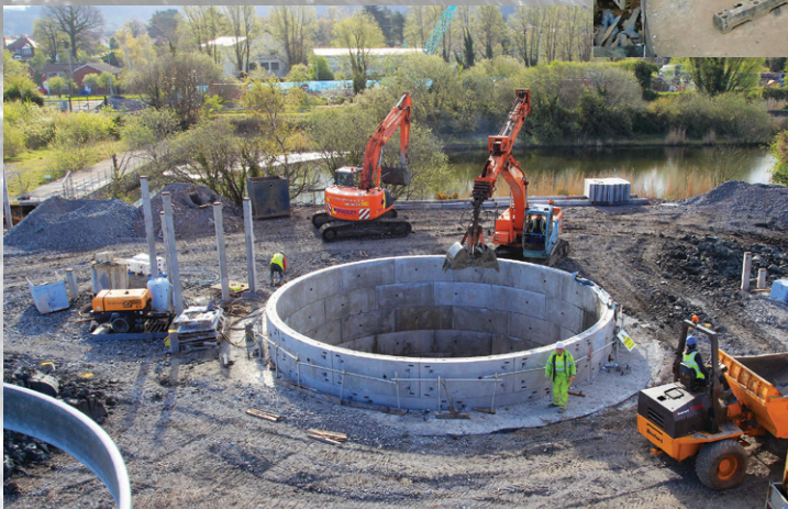
(Foreground) new dual foul and storm water pumping station under construction (background) existing lagoons Courtesy of NI Water
