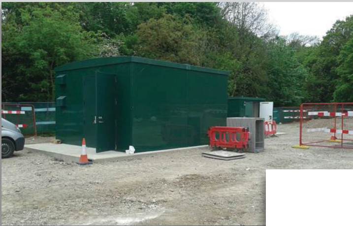
Construction of ASR3 Booster pump kiosk Courtesy of Mott MacDonald
