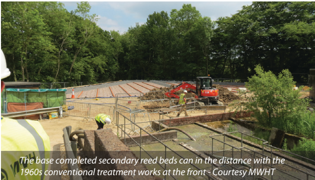
The first primary reed bed distribution pipework being installed Courtesy of MWH Treatment
