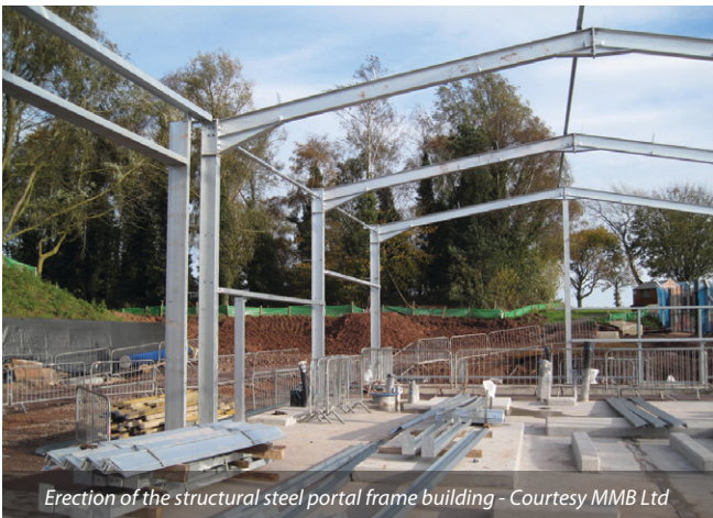
Erection of the structural steel portal frame building - Courtesy MMB Ltd
