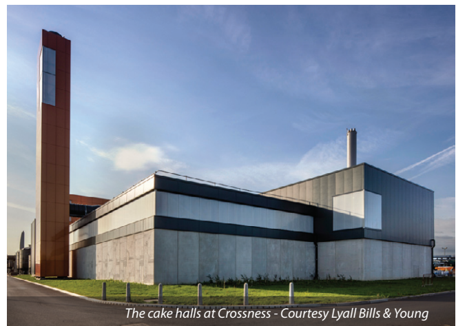
Crossness sludge cake building - Courtesy Lyll Bills & Young
