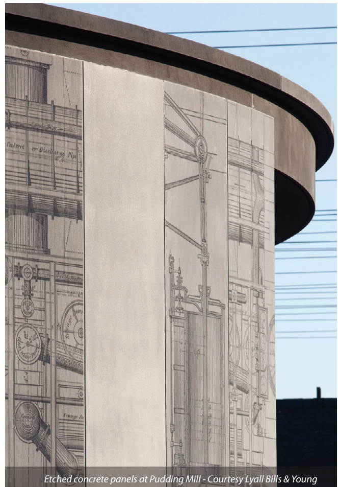
Pudding Mill Pumping Station Odour Stack - Courtesy Lyall Bills & Young
