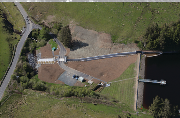
New spillway at Penwhapple Reservoir - Courtesy of LOR
