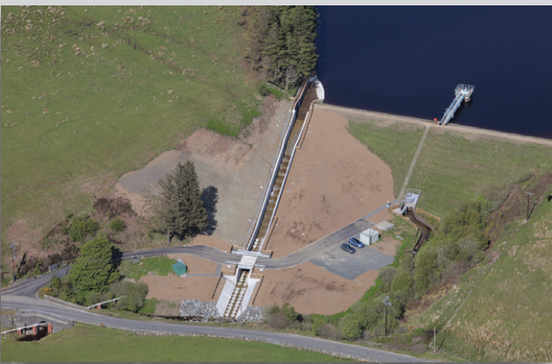
The new precast spillway at Penwhapple Reservoir - Courtesy of LOR
