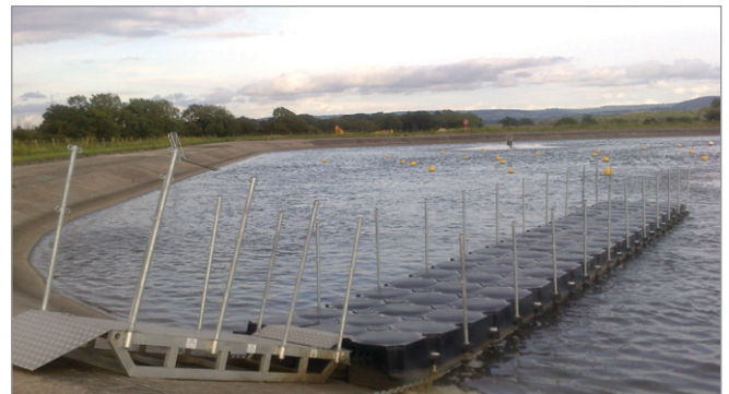
Floating Pontoon to allow inspection and greasing of motors while in situ, minimising the need to remove aerator units from the tank. Pontoon also enables attaching of crane lifting hook for removal Courtesy of Atkins
