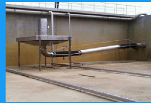
AQUA DECANT™ Floating decanter
