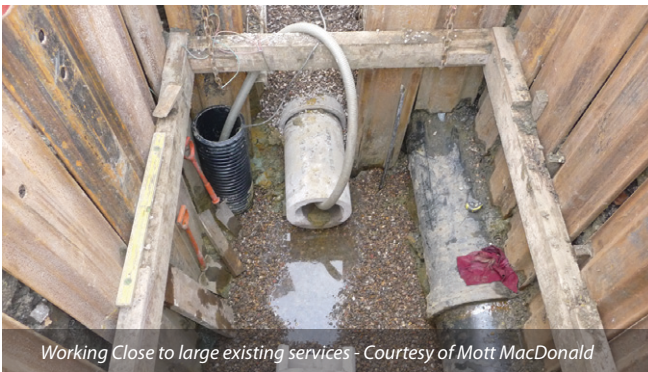
Safety on site - Courtesy of Mott MacDonald
