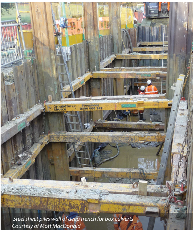
Working Close to large existing services - Courtesy of Mott MacDonald
