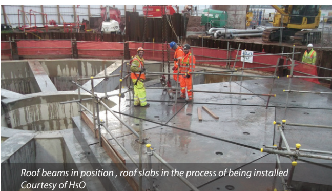
All roof beams in place - Courtesy of H5O
