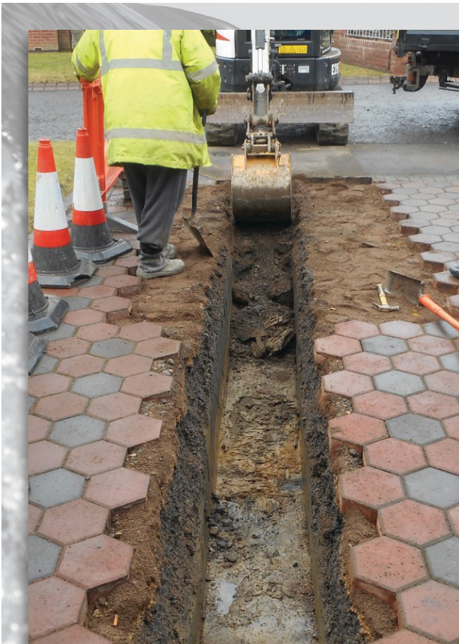
Block paving removal exposing the existing pipework - Courtesy Grontmij
