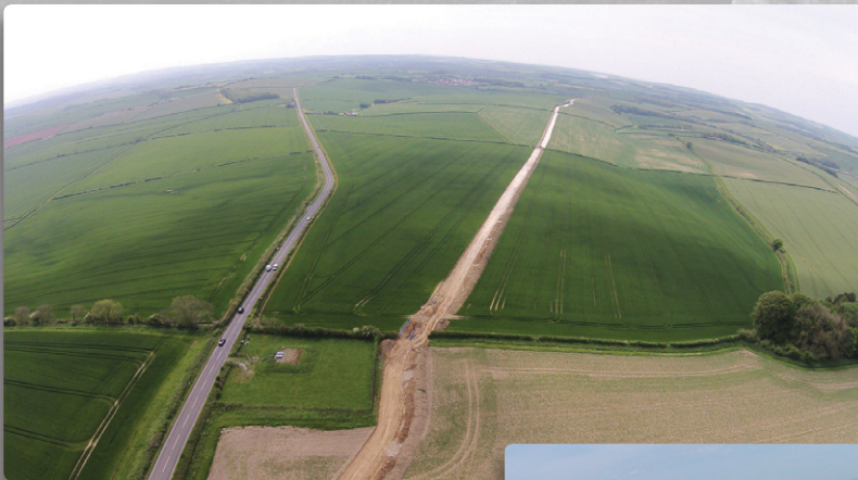
Forston to St Catherines pipeline Courtesy of Wessex Water
