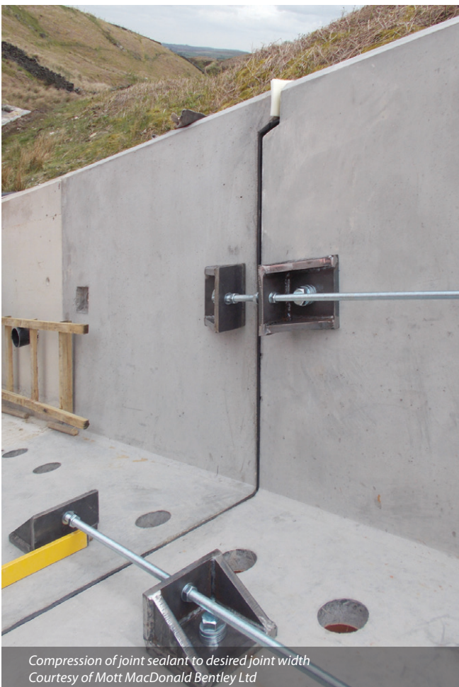
Spillway rail system installation Courtesy of Mott MacDonald Bentley Ltd
