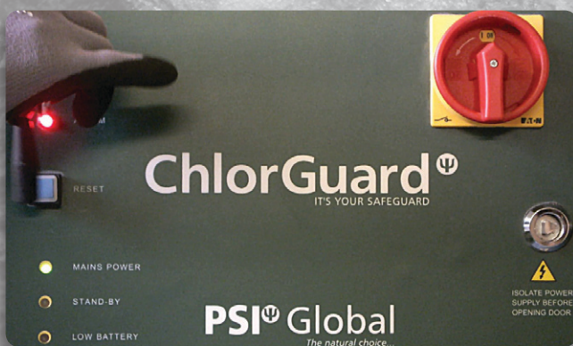
System is activated by sensor or external shut off points
