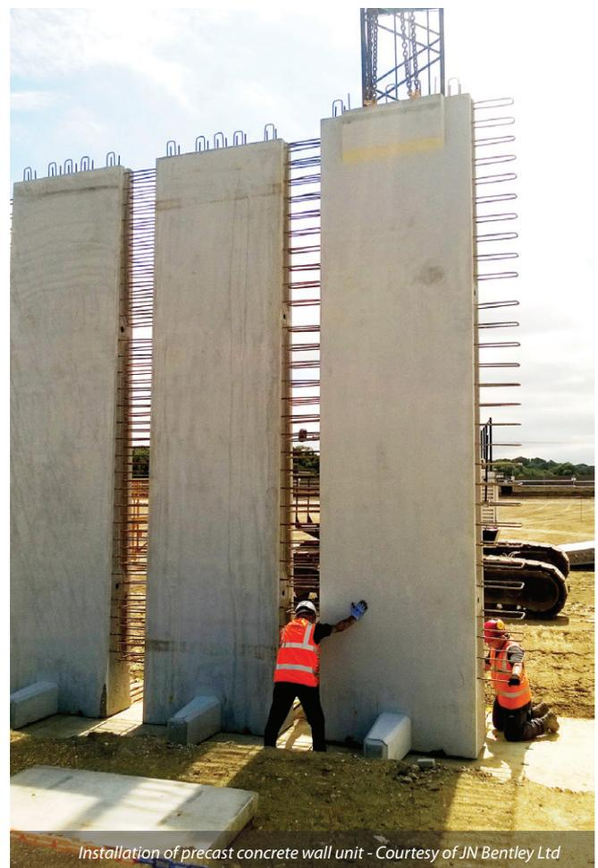
Installation of precast concrete wall unit - Courtesy of JN Bentley Ltd
