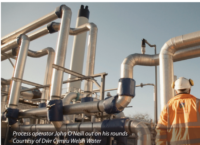
(Foreground) Five Fords Solar Ph 2 and (background) tankers delivering sludge for the digester plant - Courtesy of Dŵr Cymru Welsh Water
