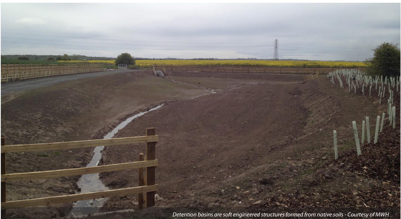
*Detention basins are soft engineered structures formed from native soils - Courtesy of MWH*
