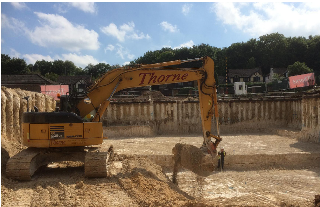
Phase 1 Excavation for the RGF Building at Woodmansterne WTW
