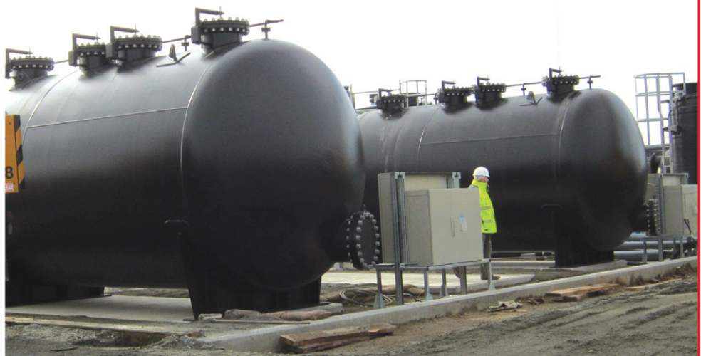
GAC & Pressure Filter Vessels used in Guernsey Airport Water Treatment Facility Project DESIGNED & MANUFACTURED BY PRESSVESS
