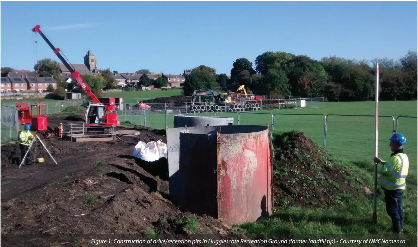
Figure 1: Construction of drive/reception pits in Hugglescote Recreation Ground (former landfill tip) - Courtesy of NMCNomenca
