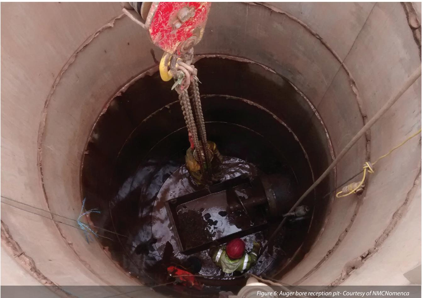
Figure 6: Auger bore reception pit- Courtesy of NMCNomenca
