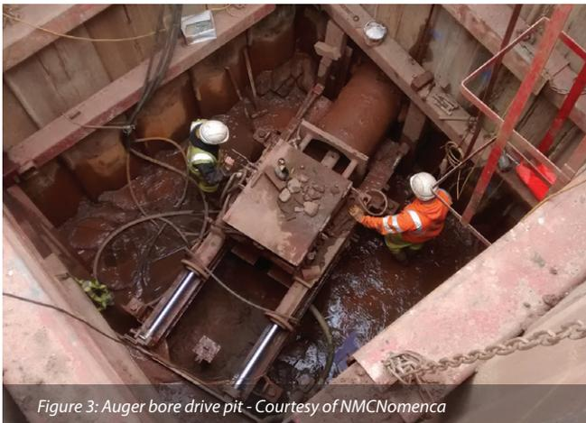
Figure 3: Auger bore drive pit – Courtesy of NMCNomenca
