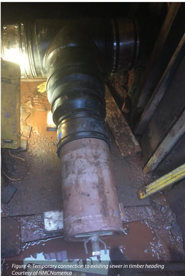
Figure 4: Temporary connection to existing sewer in timber heading
