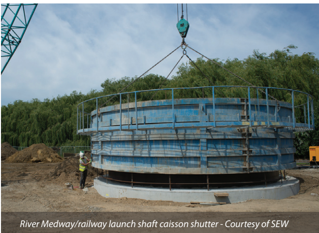
River Medway/Railway launch shaft construction - Courtesy of SEW
