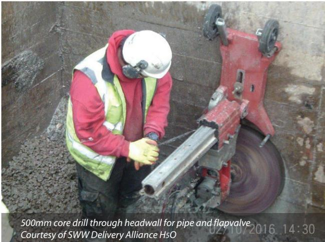
500mm core drill through headwall for pipe and flapvalve
