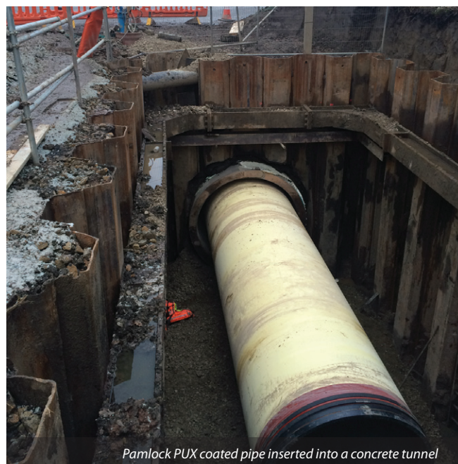
1200mm diameter Universal PUX twin main
