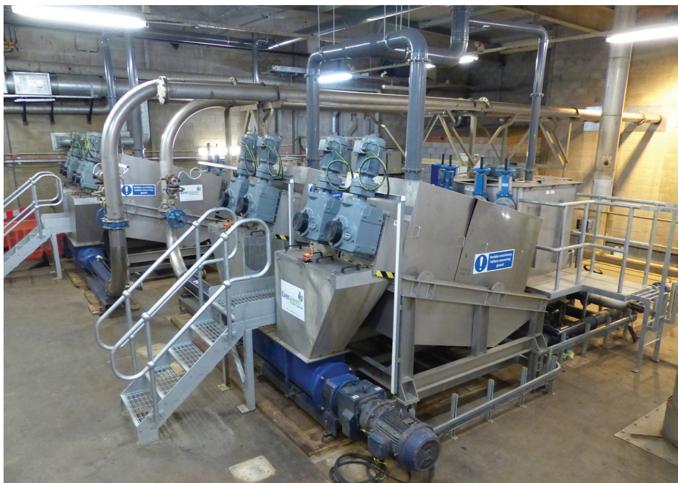
The installation of 2 (No.) ES354 Volute units (a total of eight drums) in operation shortly after commissioning - Courtesy of KWS Grampian
