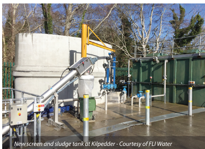
Sludge return pipework at Kilpedder - Courtesy of FLI Water
