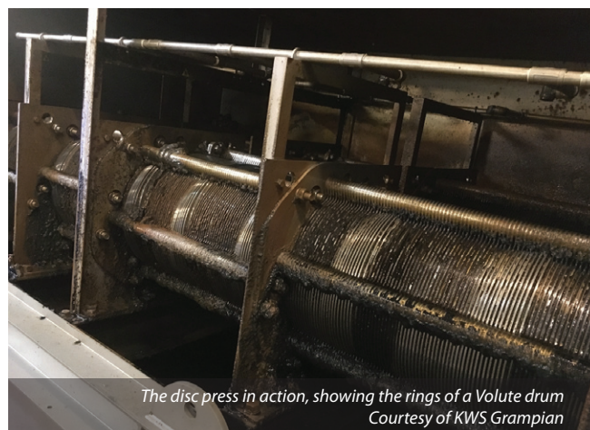
What a comparison! Looking across the area where the belt presses stood towards the Volute machines - Courtesy of KWS Grampian
