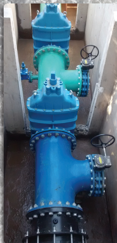
Pipework in a newly extended existing chamber ready for the new UV plants in and outlets Courtesy of NMCNomenca
