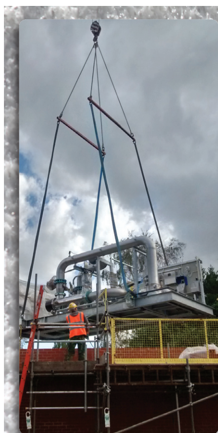
Lifting the factory built UV disinfection rig in to the new building Courtesy of NMCNomenca
