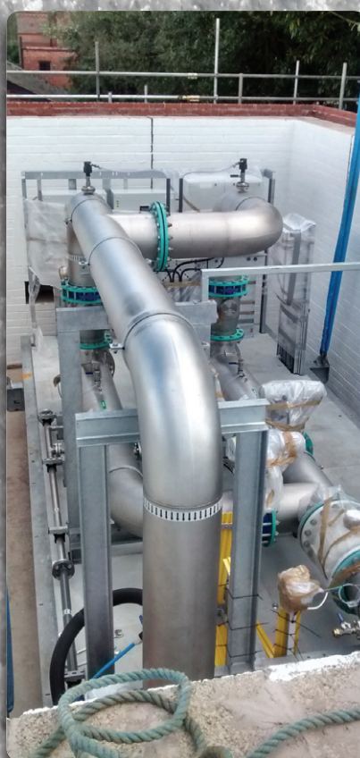
UV factory built assembly in final location. UV FBA built by Lintott Control Systems Ltd Courtesy of NMCNomenca
