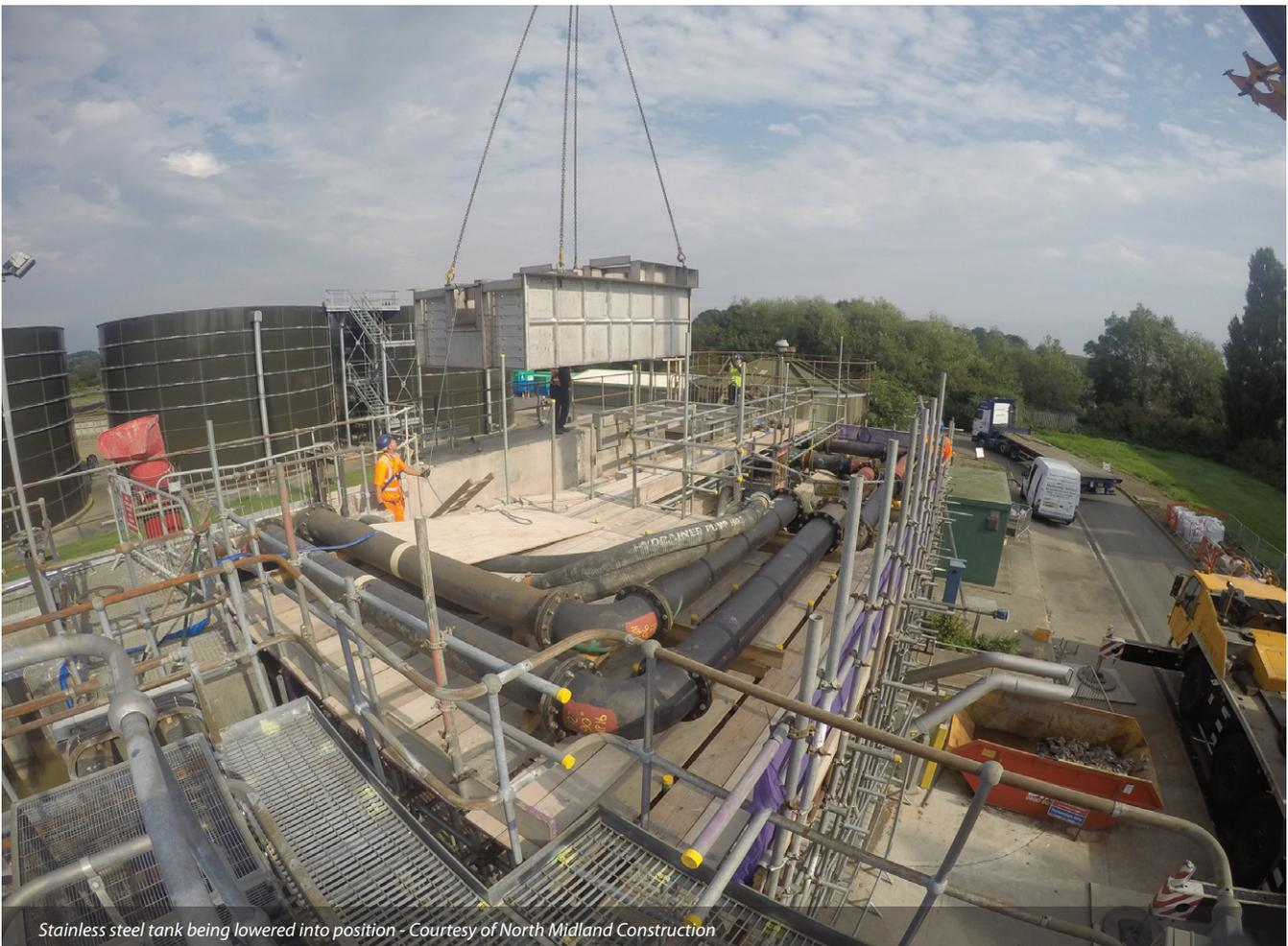
Stainless steel tank being lowered into position - Courtesy of North Midland Construction
