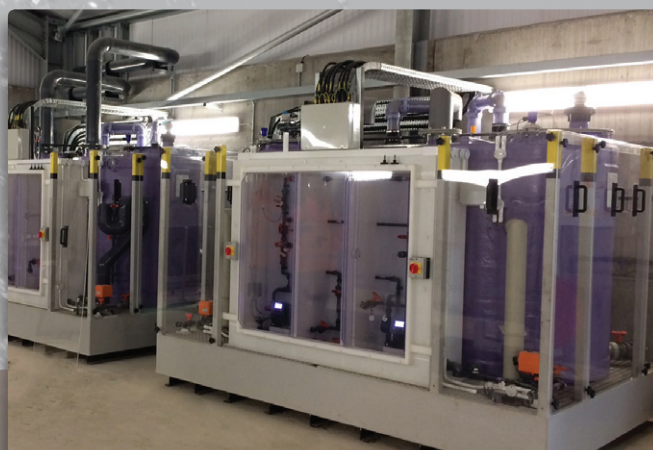
Antiscalant and hypochlorite dosing rigs Courtesy of MMB
