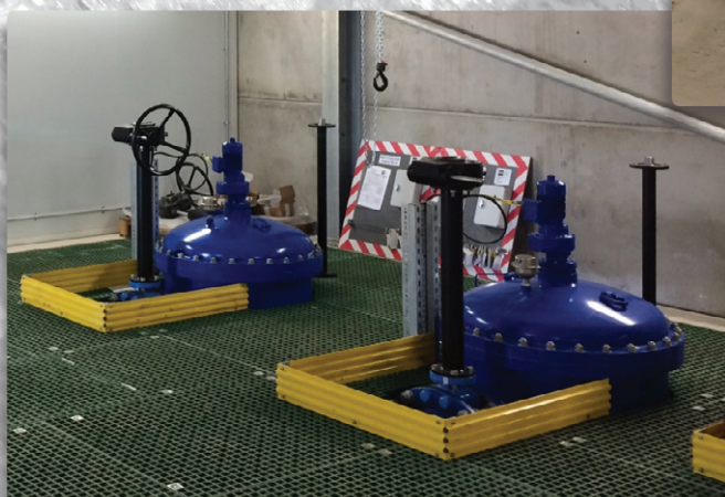
Bollfilters and lifting equipment Courtesy of MMB
