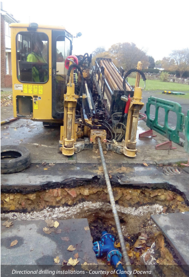
Construction underway - Courtesy of Southern Water
