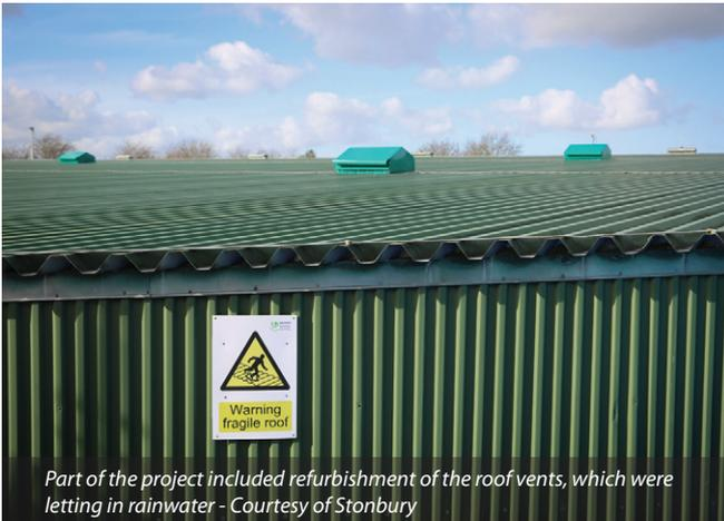
Part of the project included refurbishment of the roof vents, which were letting in rainwater - Courtesy of Stonbury
