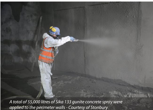
A total of 55,000 litres of Sika 133 gunite concrete spray were applied to the perimeter walls - Courtesy of Stonbury
