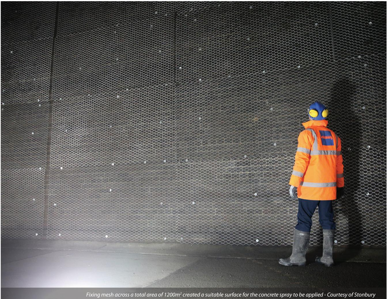
*Fixing mesh across a total area of 1200m<sup>2</sup> created a suitable surface for the concrete spray to be applied - Courtesy of Stonbury*
