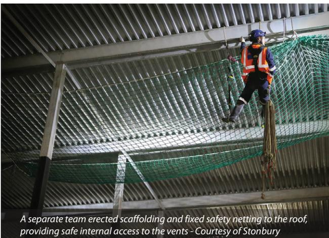
A separate team erected scaffolding and fixed safety netting to the roof, providing safe internal access to the vents - Courtesy of Stonbury
