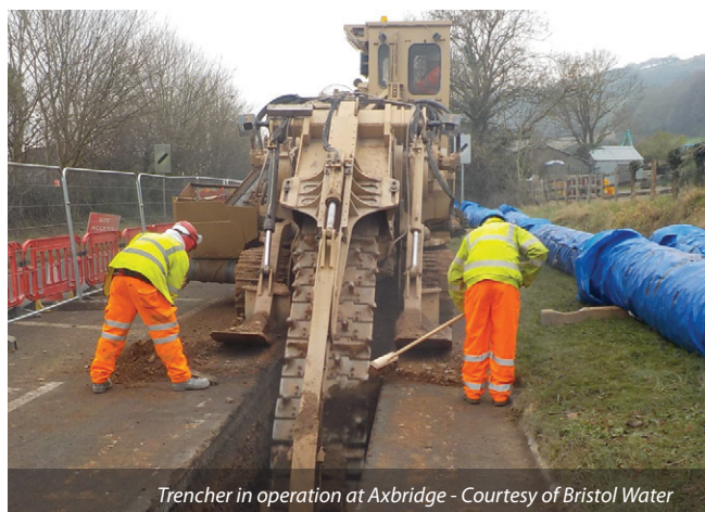
Stringing of ductile iron pipe near Axbridge - Courtesy of Bristol Water
