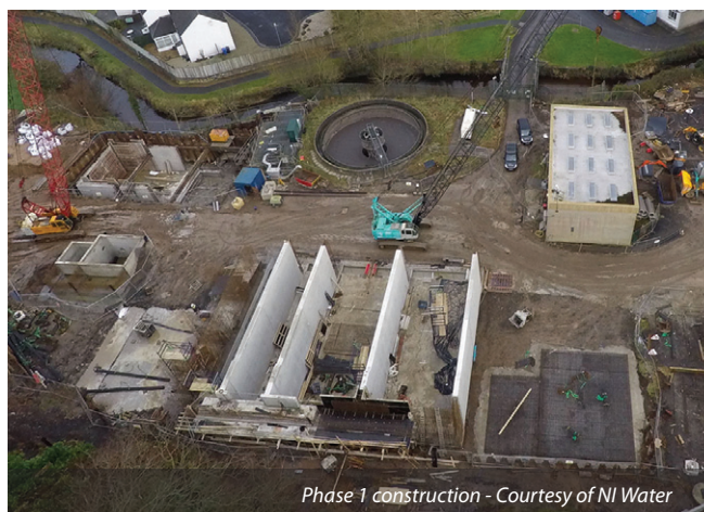
Storm tanks 440m 3 concrete pour - Courtesy of NI Water
