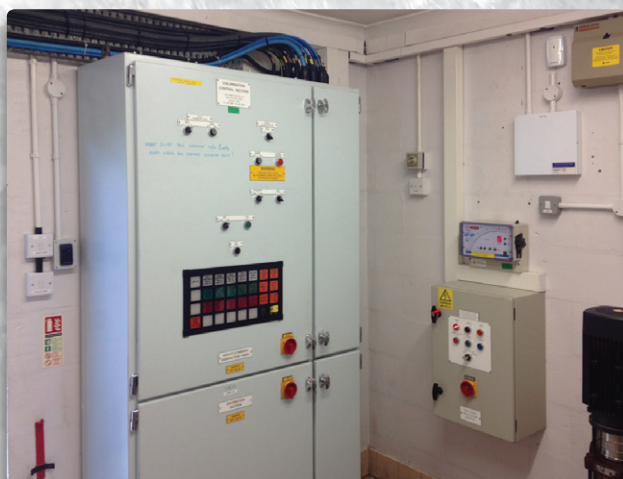
Chlorination panel - Courtesy of Severn Trent Water
