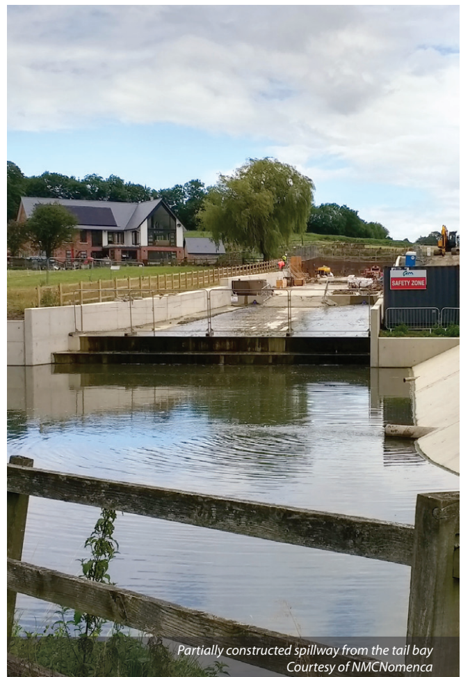
Construction underway - Courtesy of NMCNomenca
