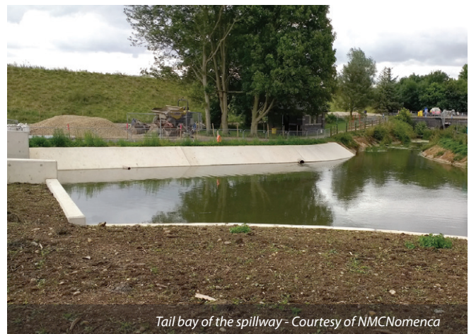
Partially constructed spillway from the tail bay Courtesy of NMCNomenca
