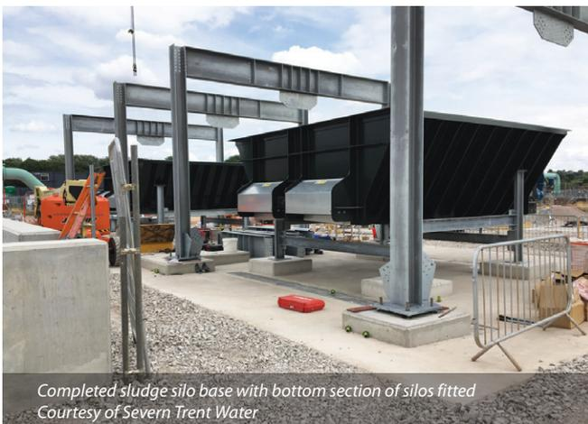
Completed sludge silo base with bottom section of silos fitted
