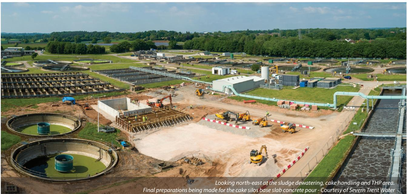
Looking north-east at the sludge dewatering, cake handling and THP area. Final preparations being made for the cake silos base slab concrete pour - Courtesy of Severn Trent Water
