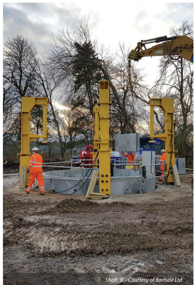
MTBM at Shaft 'B' - Courtesy of Barhale Ltd
