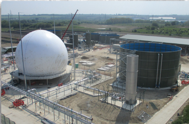
General view over Area Y under construction - Courtesy of YWS
