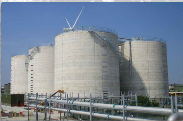
General view of digester compound under construction - Courtesy of YWS
