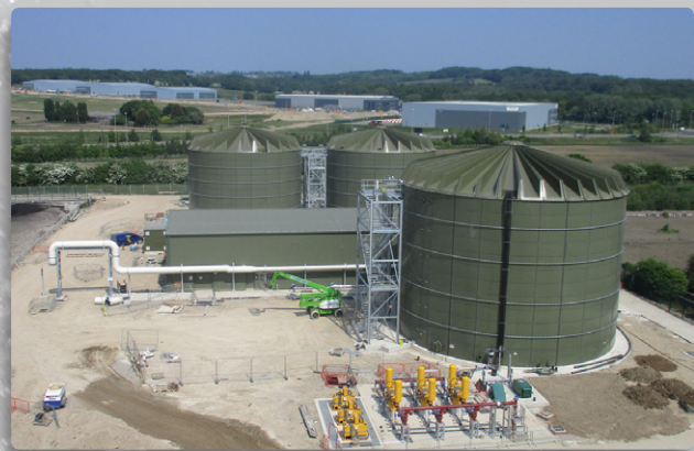
Sludge thickening process area under construction - Courtesy of YWS
