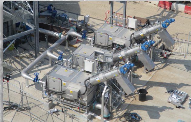
Liquid imports sludge screens under construction - Courtesy of YWS
